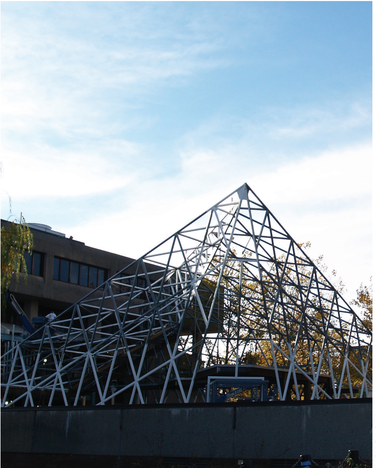
Student Union Building addition under construction.
